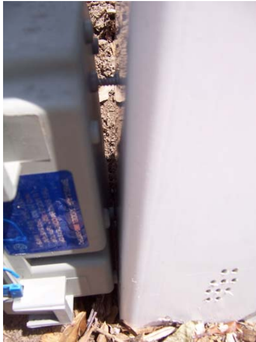
Figure 14. Pictures of the inside of an empty pump tank attached to a functioning FAST system. The installer indicated that a plug at the bottom of the tank came out and has encountered this problem at other sites.
