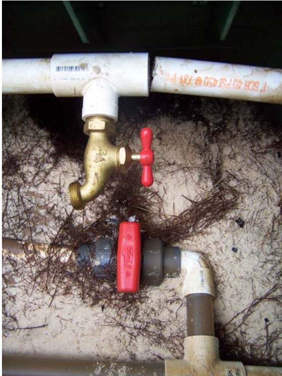
Figure 17. Pictures of site WS-4 taken on April 14, 2009. The broken plumbing evident in this picture was also reported in September 2008. The broken pipe causes the effluent to fill the control box instead of going to the drain field.
