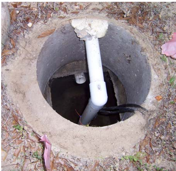
Figure 14. Pictures of the inside of an empty pump tank attached to a functioning FAST system. The installer indicated that a plug at the bottom of the tank came out and has encountered this problem at other sites.
