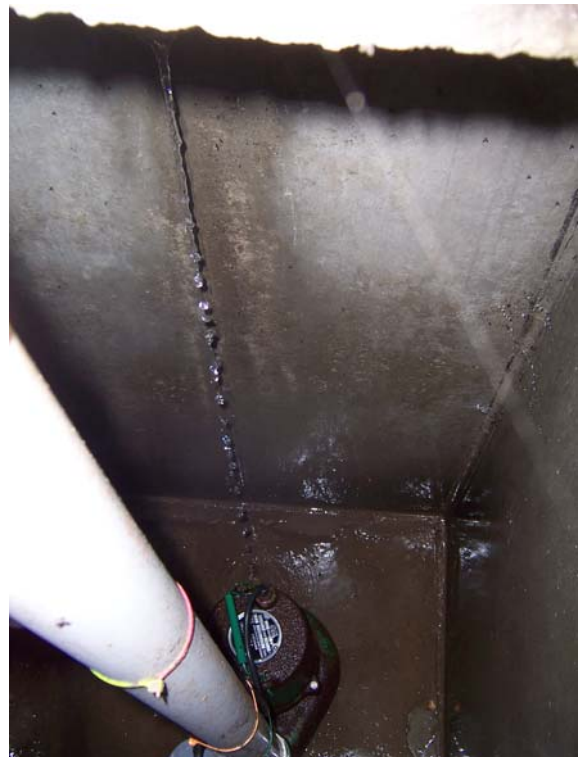
Figure 14. Pictures of the inside of an empty pump tank attached to a functioning FAST system. The installer indicated that a plug at the bottom of the tank came out and has encountered this problem at other sites.
